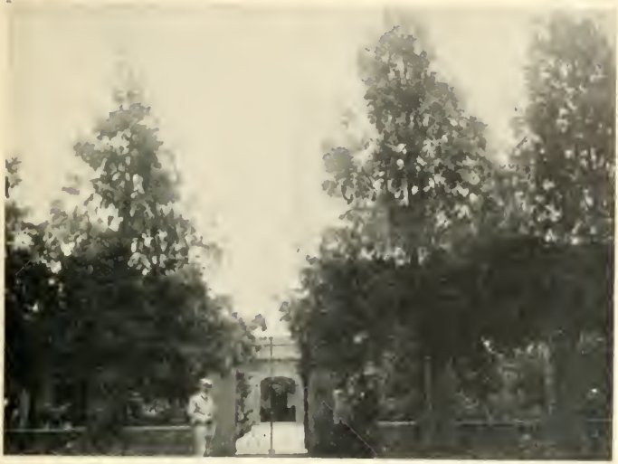
BICHADERO ESTANCIA—ENTRANCE TO COURTYARD.
